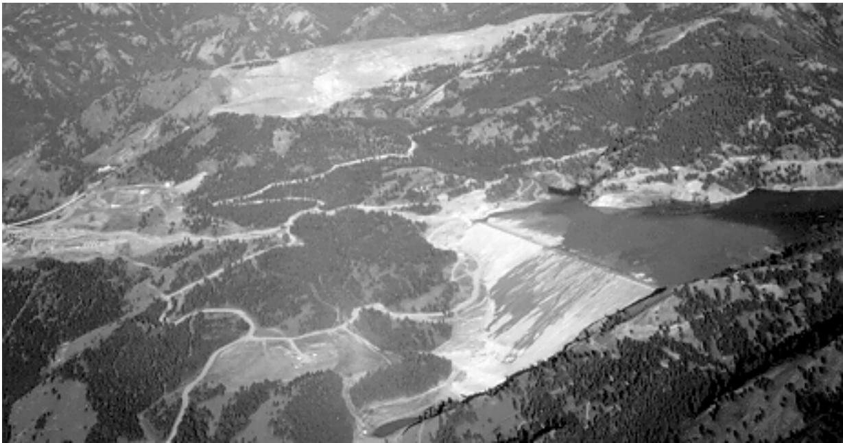
Tailings Pond and Dam (Foreground) and Pit and Mill at the Thompson Creek Mine, a molybdenum mine near Clayton, Idaho. Streaks on the dam face are tailings being deposited on the dam face to raise the level of the dam.
