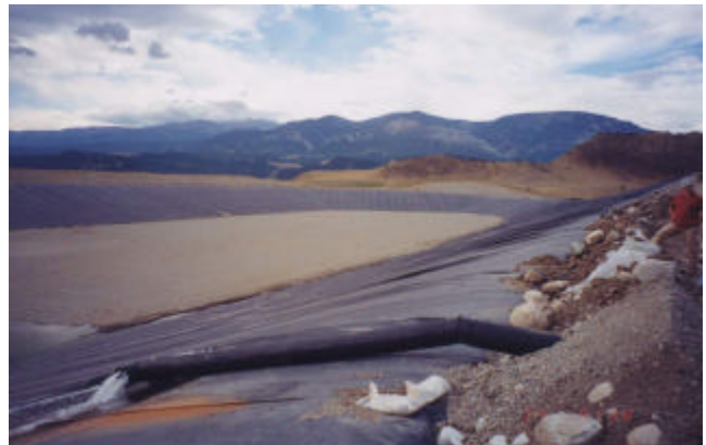
Hertzler Tailings Impoundment under construction
