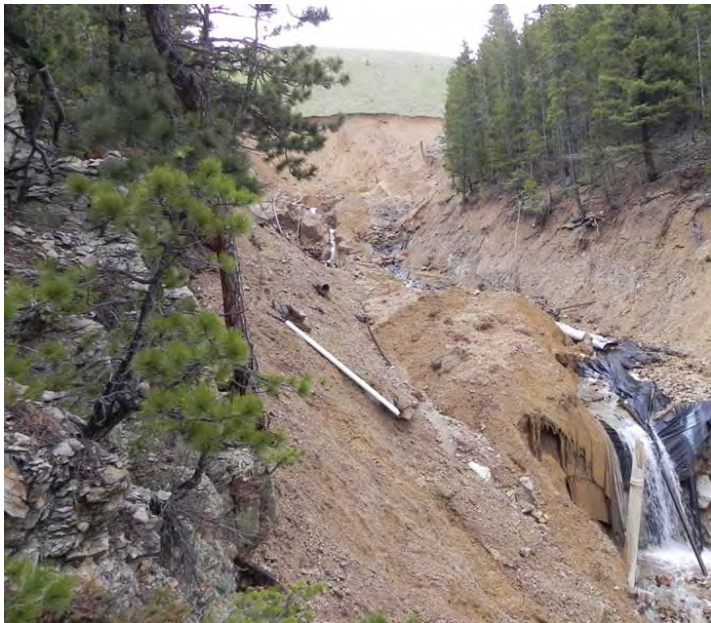
Alder Gulch Waste Dump failure at the Zortman Mine
