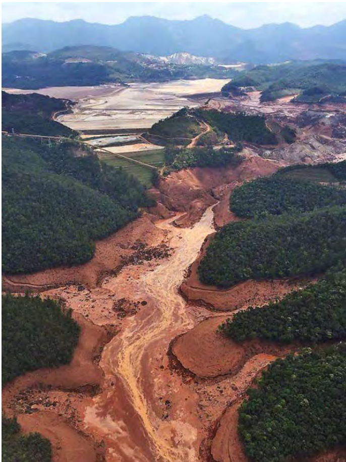
Fundao Tailings Dam Failure, Brazil, November 2016
