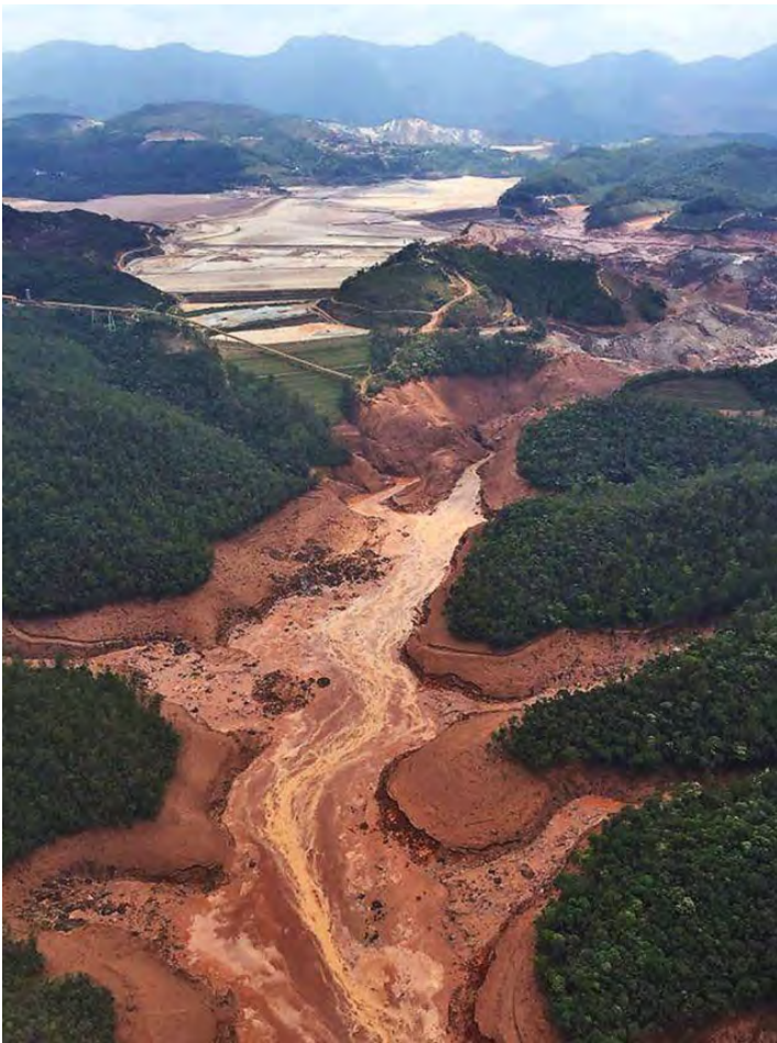
Fundao dam failure, Brazil, November 5, 2015
