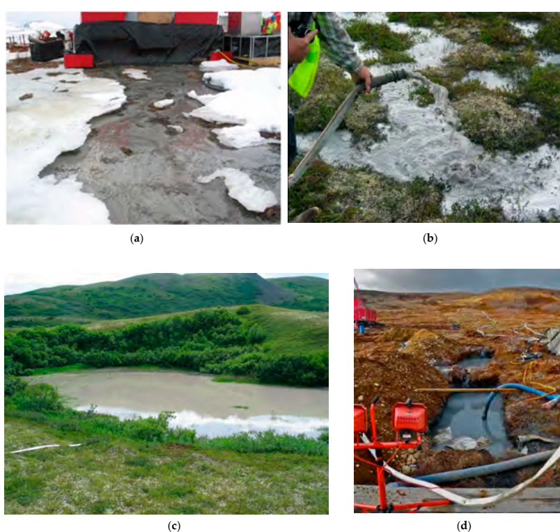
Figure 2. Drill waste discharged to land. (a) Direct discharge of drill waste, including drill cuttings. (b) Discharge of sump water. (c) Disposal of drill waste to kettle depression. Source: [4,5]. (d) Drill waste sump. Note that all waste sumps were unlined. Photo credit: M. Welker.
