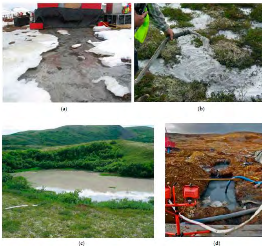
Fig. 2. Drill waste discharged to land. (a) Direct discharge of drill waste, including drill cuttings. (b) Discharge of sump water. (c) Disposal of drill waste to kettle depression. Source: [6,7]. (d) Drill waste sump. Note that all waste sumps were unlined
