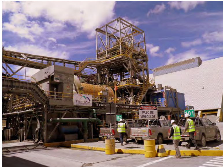
Figure 12 Portion of Tintaya's Current Processing Facility (Mill)
