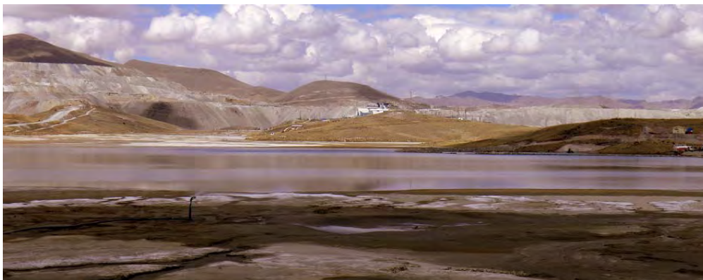
Figure 7 One of Tintaya's Current Tailings Disposal Areas (Ponds)
