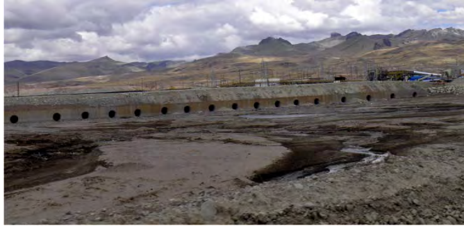
Figure 4 Canipia River Flow-Thru at Antapaccay Mine Site
