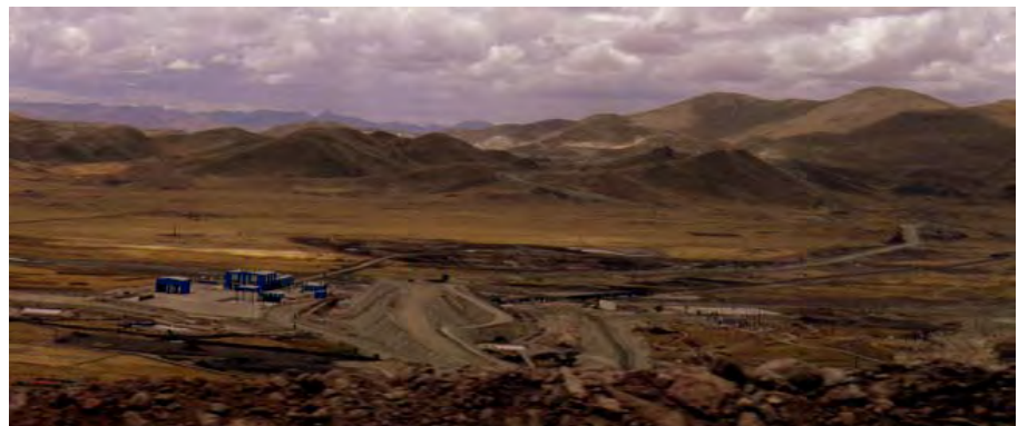
Figure 11 Antapaccay Mine Loading Facility and Conveyor Belt
