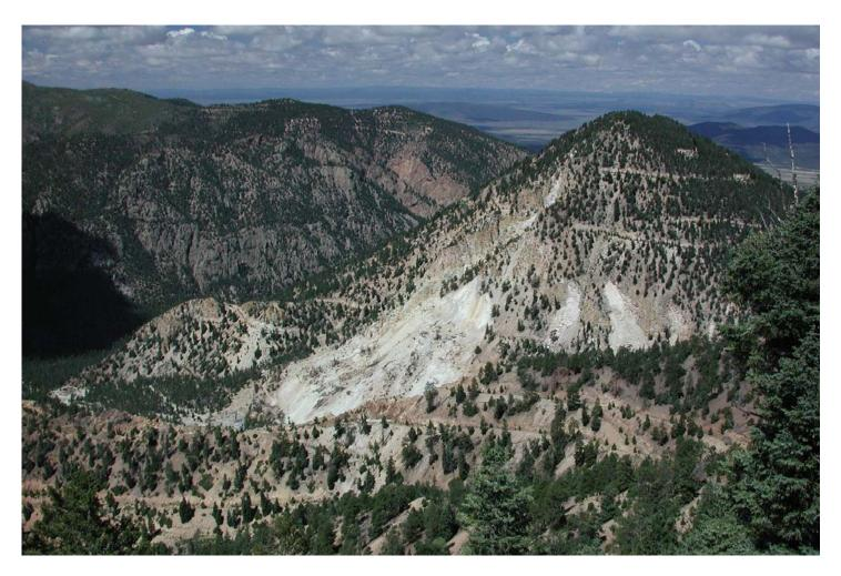
Surface subsidence scarp (white area) formed along fault plane on Goat Hill. Scarp is caused by underground block-cave mining at the Molycorp mine (October 2001).
